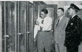
New auxiliary station operates four 250-watt transmitters, two channels for police, two for fire.
